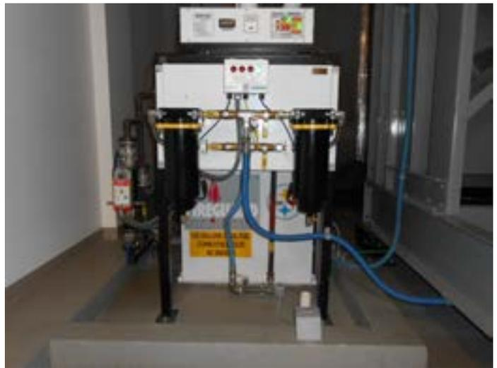
48. 100-gallon fuel oil storage tank with secondary containment structure on second floor Phase I section of Dupont Fabros Technology building.
