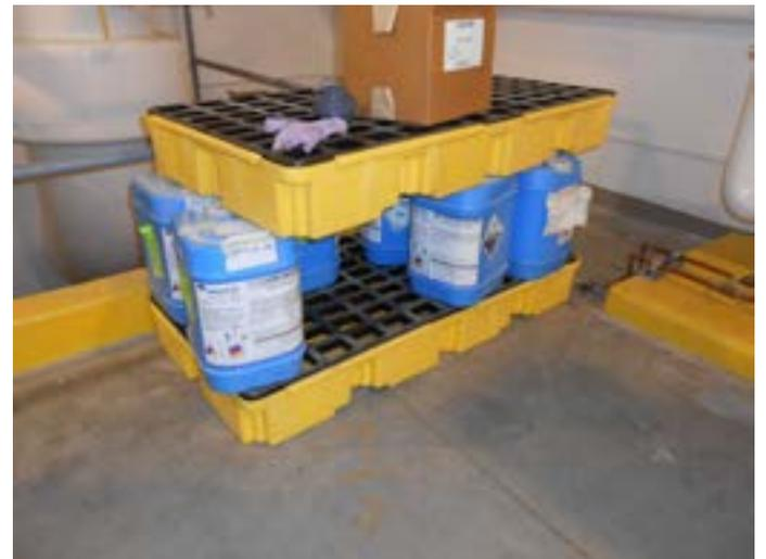
60. 5-gallon containers of defoaming agent for chiller system in Chiller Room in Phase II section of DuPont Fabros Technology Building.
