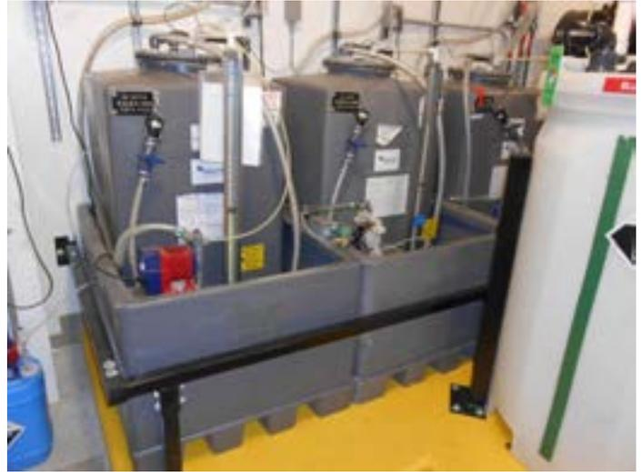
58. Storage tanks of water treatment solution with secondary containment structures in Phase II section of DuPont Fabros Technology Building.
