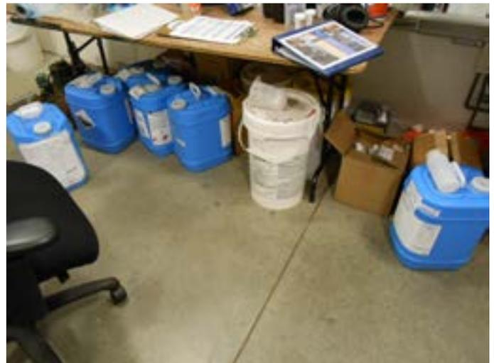
56. 5-gallon containers of defoaming agent for chiller system and 50 pound container of Towerbrom brand microbiocide in Chiller Room in Phase I section of DuPont Fabros Technology Building.
