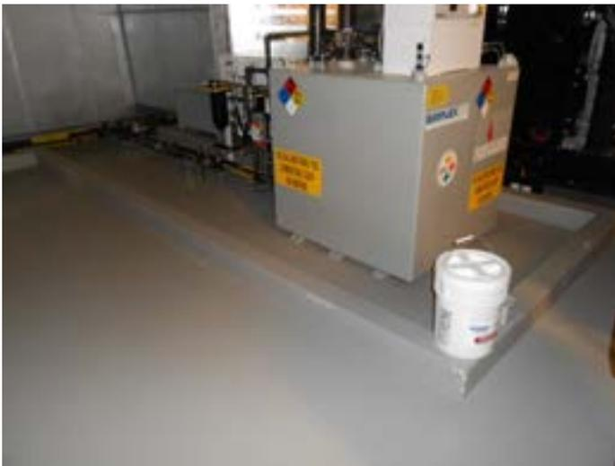
51. 100-gallon fuel oil storage tank with secondary containment structure on second floor of Phase II section of DuPont Fabros Technology building.
