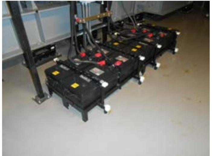
50. Lead-acid batteries connected to emergency power generator on second floor of Phase I section of DuPont Fabros Technology building.
