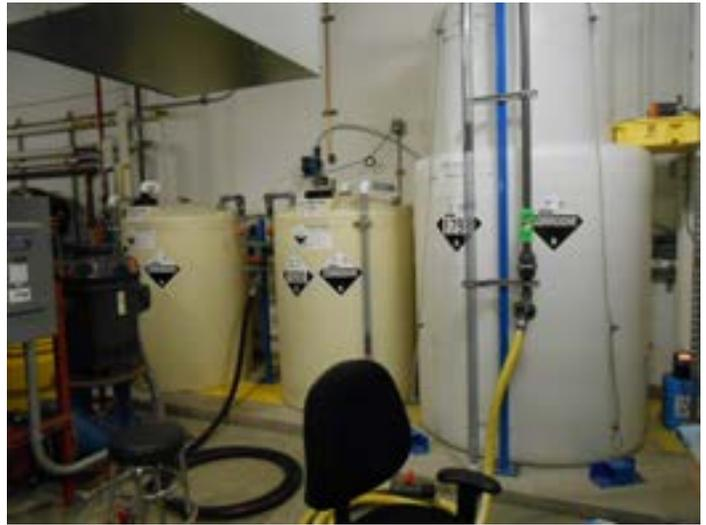
54. Two 405-gallon storage tanks containing sulfuric acid and one 1,000 gallon storage tank containing sodium hypochlorite in Chiller Room in Phase I section of DuPont Fabros Technology Building.
