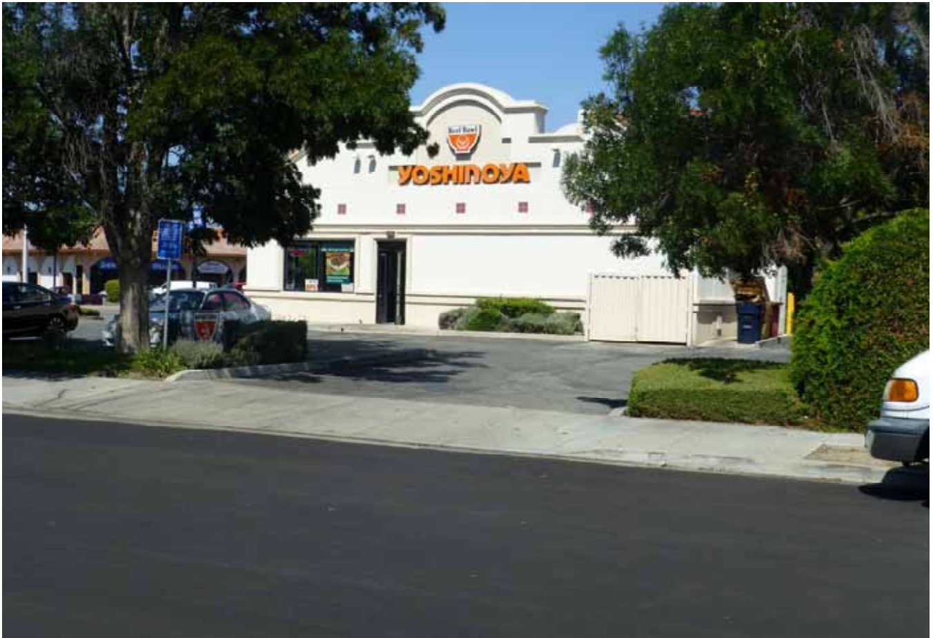
15. View of restaurant to the east across Pierce Street.
