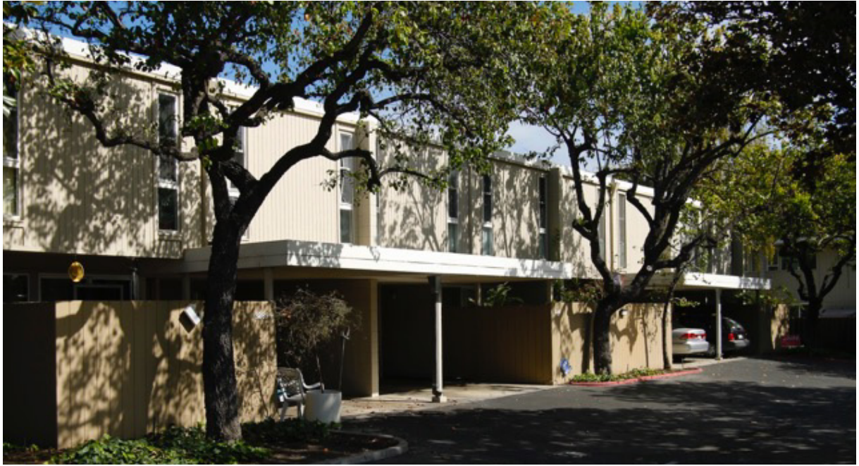
a) Multi-family residences immediately south of project site
