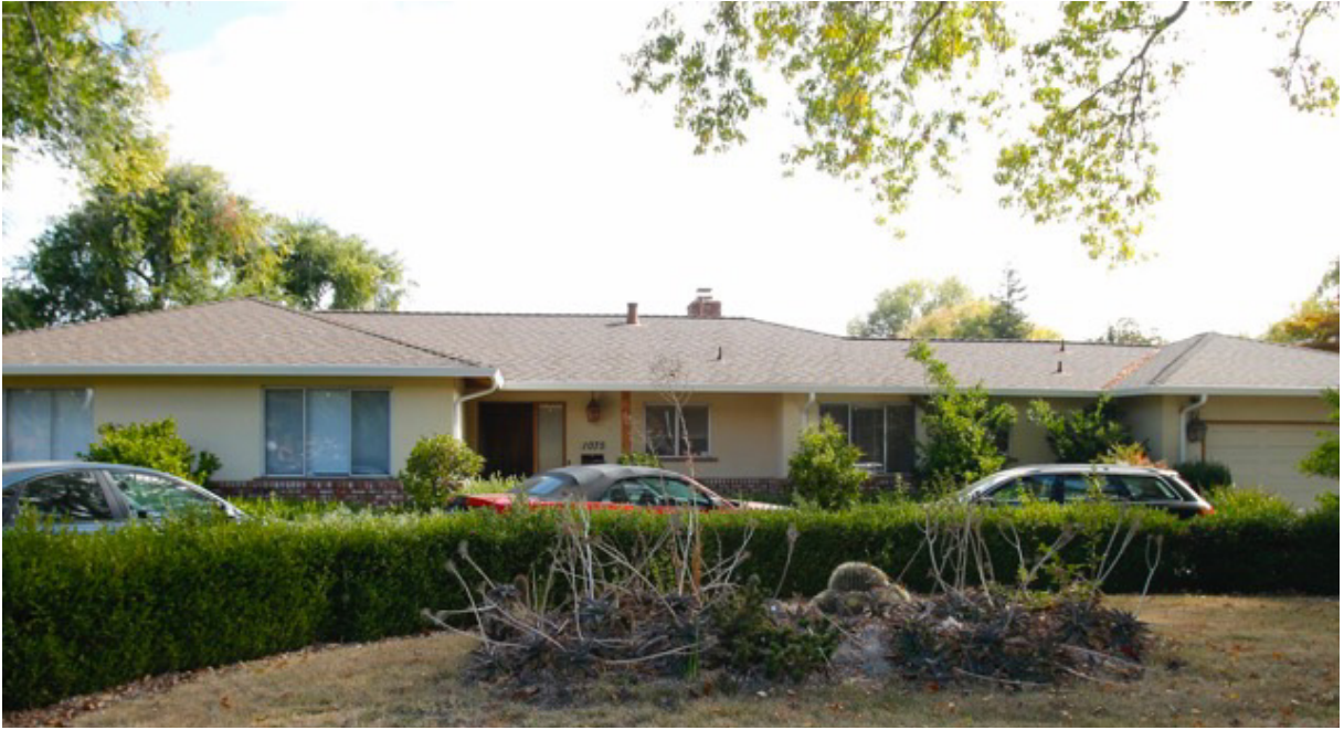
a) Existing conditions at 1075 Pomeroy Avenue
