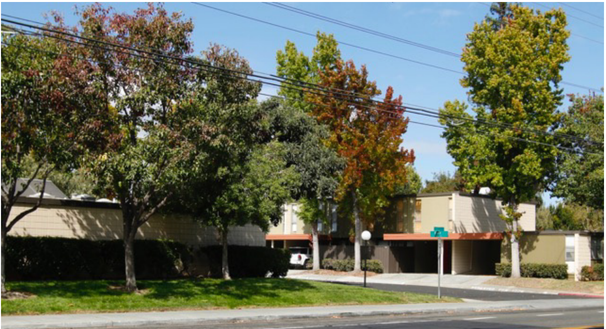
b) Existing conditions immediately west of the project site
