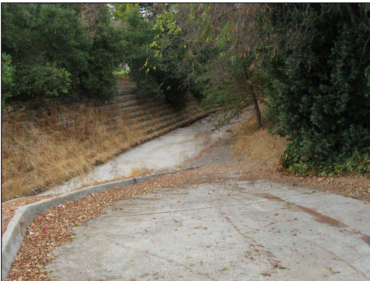
A SCVWD maintenance access ramp is located on the southwest corner of Homestead Road. Access to the channel bed must be retained. SCVWD access is also available at Kiely Boulevard. Providing access at only one location should be further explored in the creek trail master plan.
