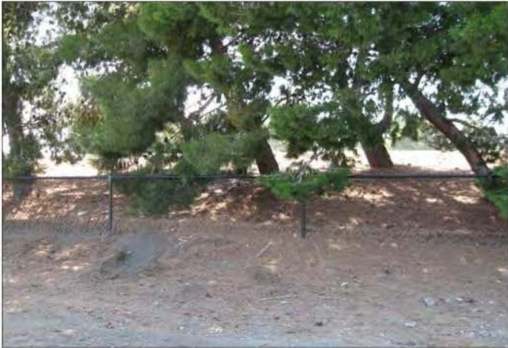
Photo 15 - View of the San Tomas Aquino Creek levee, looking west from the parking garage site.
