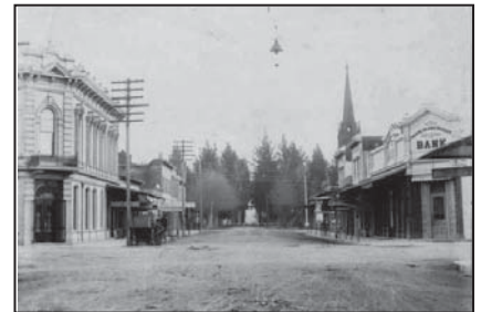
The Santa Clara Railroad Depot was constructed in 1863, and by 1916 was a bustling center of activity in the City [top and center]. The Depot, which is on the National Register of Historical Places, was the oldest continuously operated railroad depot in California until the ticket office closed in 1997. The intersection of Main Street and Franklin Street was once considered the center of Downtown Santa Clara [bottom].
