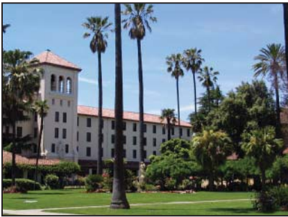
Many of Santa Clara's historic buildings, such as the Franck Mansion [top], are located in the Old Quad area. Santa Clara University continues to play an important role in the community with several public venues like Mission Santa Clara, as well as the de Saisset Museum and the Louis B. Mayer Theater [not pictured]. Nobili Hall [bottom] is a residential hall on the University campus.
