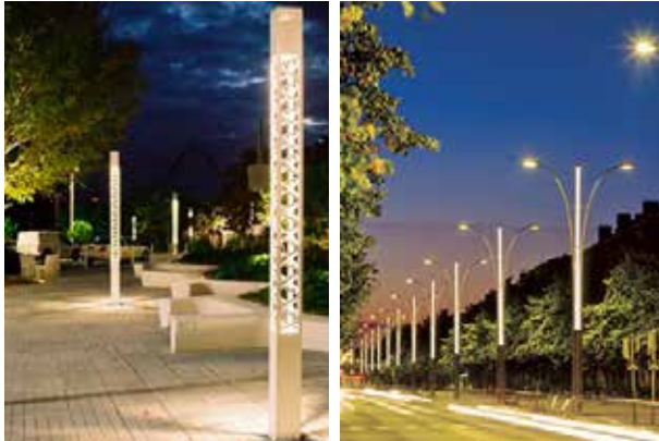
Pedestrian-scale lighting poles along sidewalks
