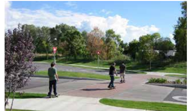
Raised crosswalk for traffic calming
