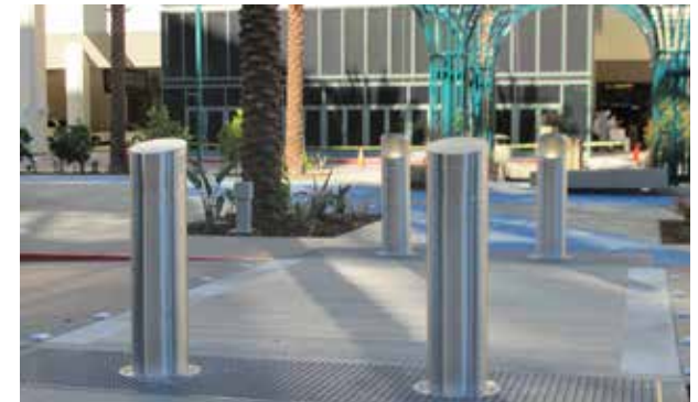
Bollards for pedestrian safety
