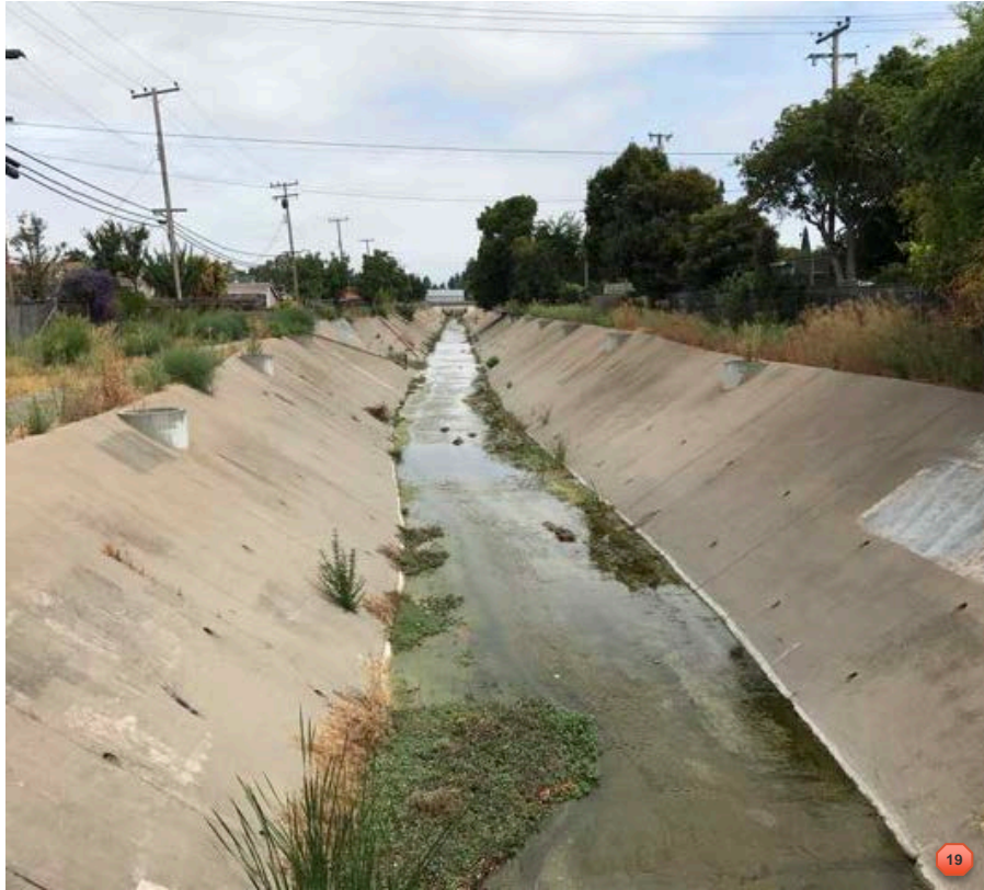
Looking downstream at Monroe toward Agate ped/bike bridge and Caltrain/JPB/UPRR corridor.
