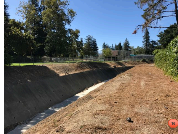
Possible ped/bike bridge location (above).
