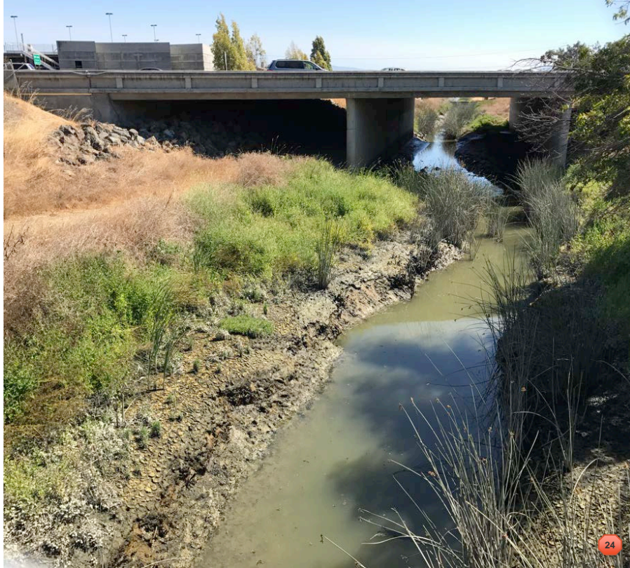
Looking upstream (south) from the Bay Trail toward Highway 237.
