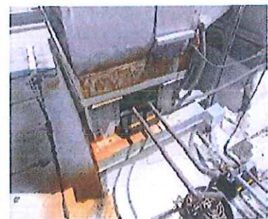
Rust at Make-Up Air Unit
