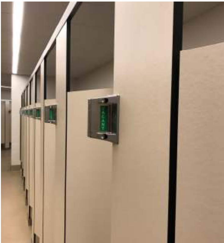
Restroom Vacancy signs
