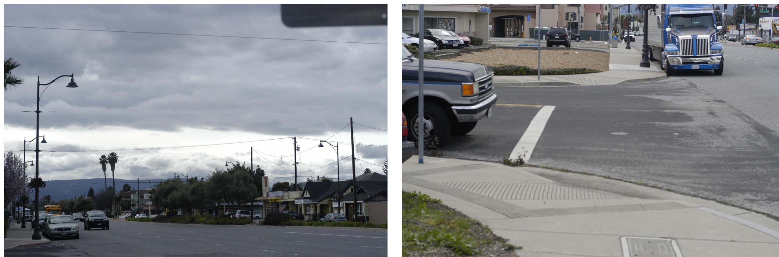
Figure 1: A (left): typical section of El Camino Real, note the width and lack of pedestrian lighting; B(right): typical sidewalk and lack of crosswalk at connection
