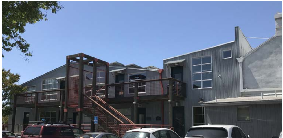
Photo: SSV office building—many windows and skylights
