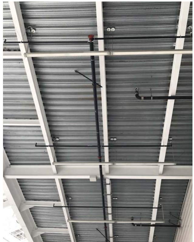
Fire Sprinkler System Upgrades
