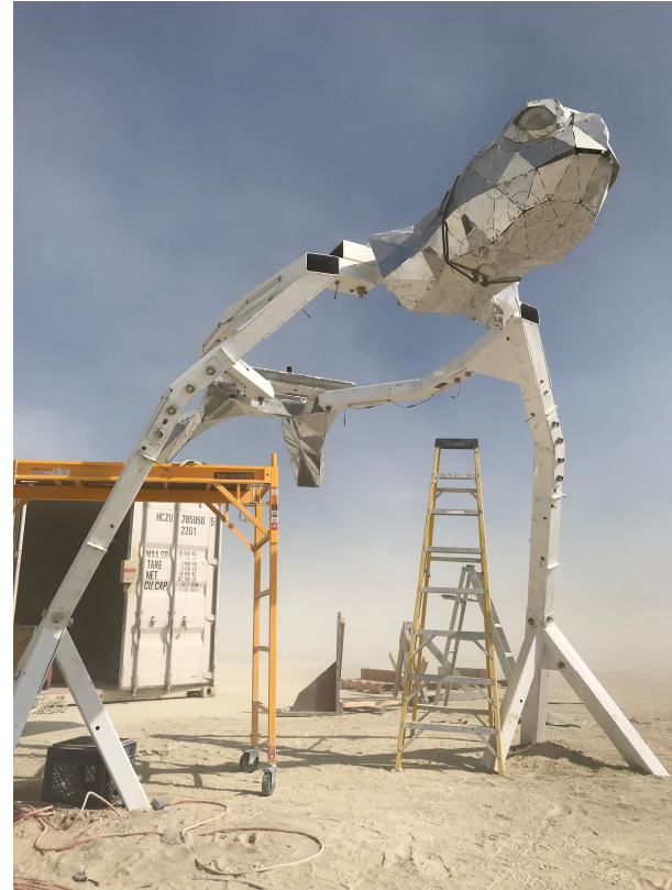
The internal frame is made from 6x4" 3/16" wall steel tubing with 1" diameter steel bolts. It is painted with corrosion resistant enamel.
