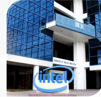
Major Data Center for Silicon Valley
