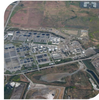
Regional Wastewater Facility
