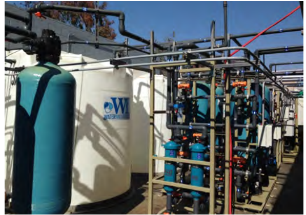
Equipment for recycling water at a local circuit board manufacturer
