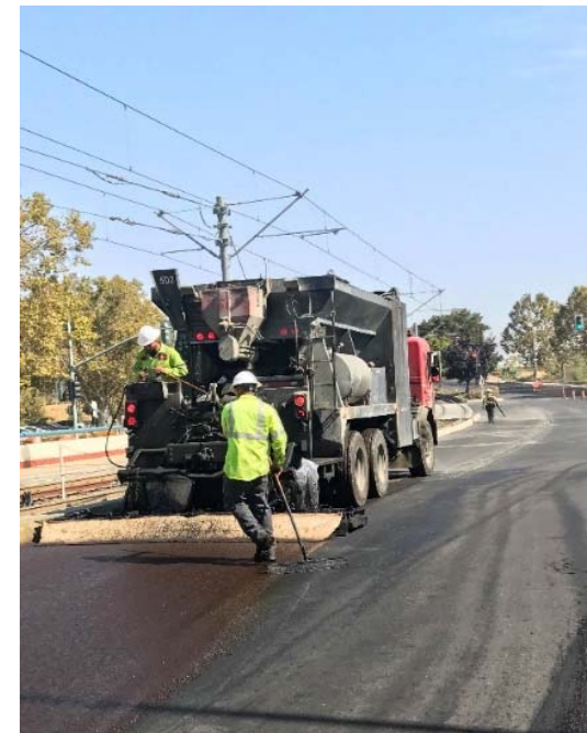
Annual Street Maintenance and Pavement Rehabilitation Program
