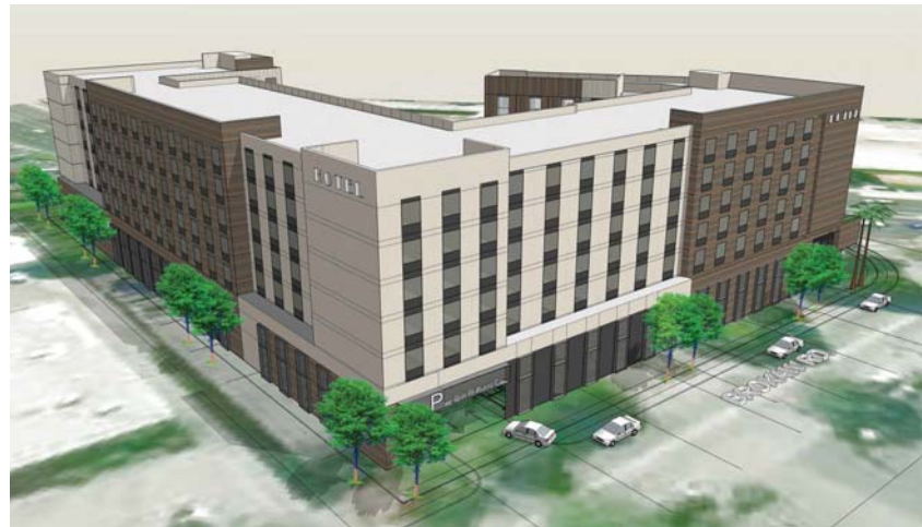
ADJACENT PROPERTY AND BROKAW ROAD
