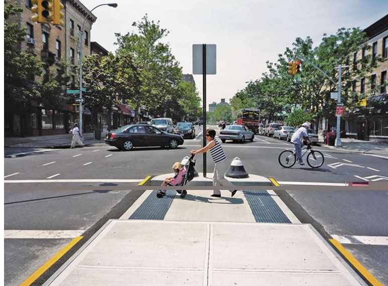
Median Refuge Island
