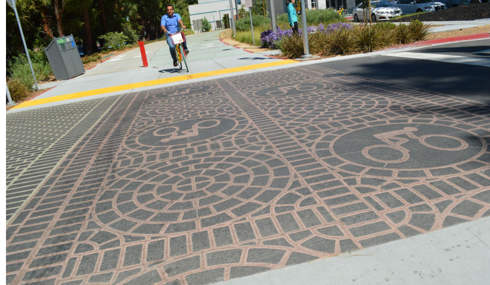
Decorative/ High-Visibility Crosswalk
