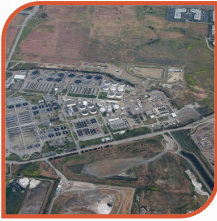
Regional Wastewater Facility*
