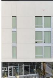
A CEMENT PLASTER
