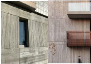
E BOARD FORMED CONCRETE
