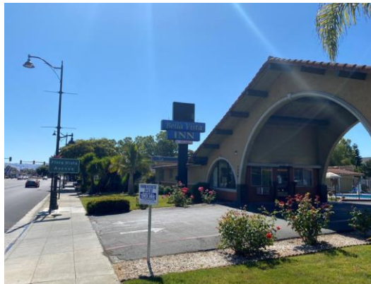
VIEW FROM EL CAMINO
