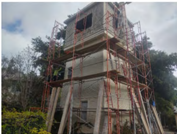
Repairs to Harris Lass
