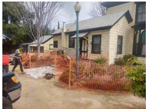
Repairs to Harris Lass
