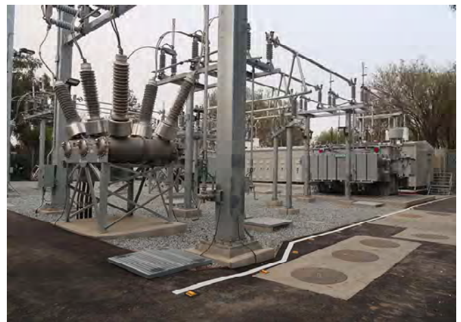
Serra Substation Rebuild
