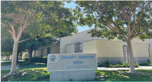
COMMUNITY RECREATION CENTER
