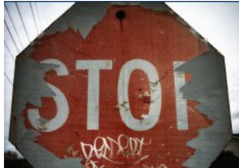
Unclear faded signage and striping
