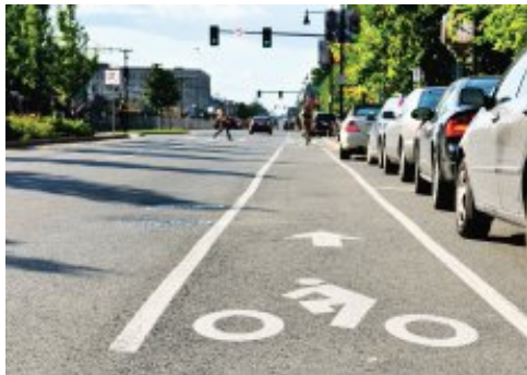
Narrow or missing bike lanes
